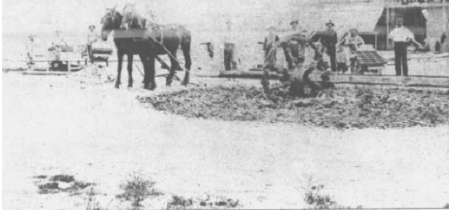
It took lots of horsepower as well as manpower to make bricks in the old days
