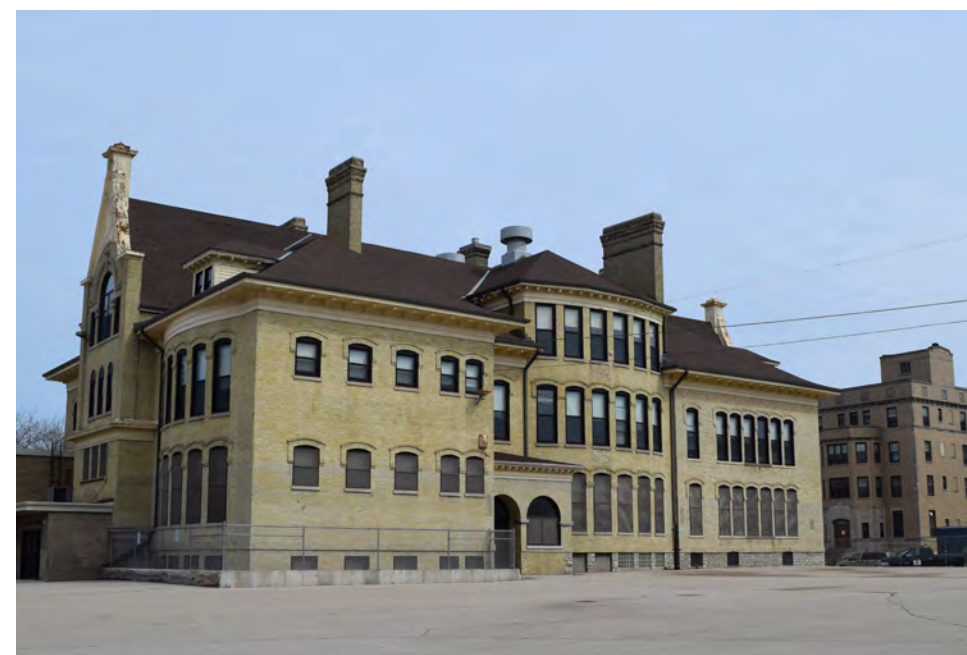
Closed Winslow Elementary School 1325 Park Avenue.
