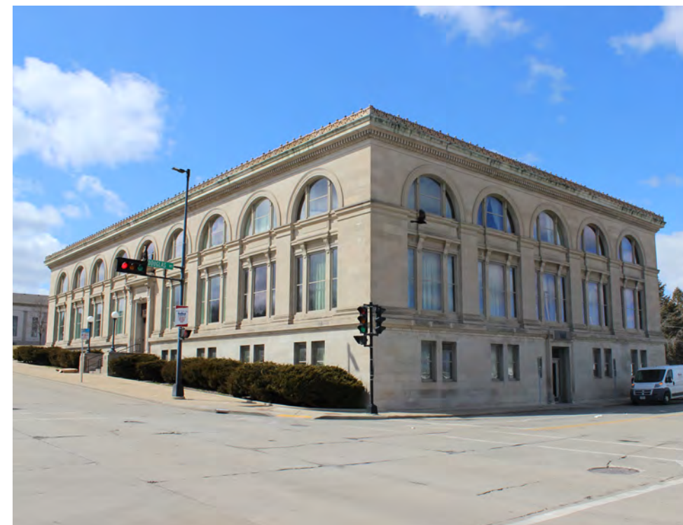
Jl Case Administration Building - 700 State Street
