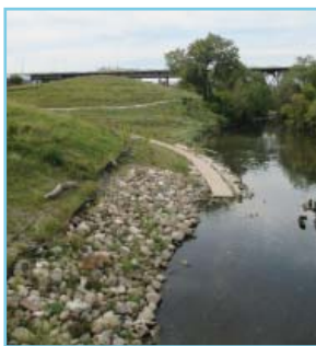
Rivers Edge Treatment and Bluff Stabilization
